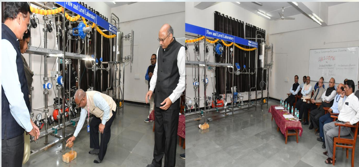
(Flow – Level Laboratory with Modern DCS Setup)
